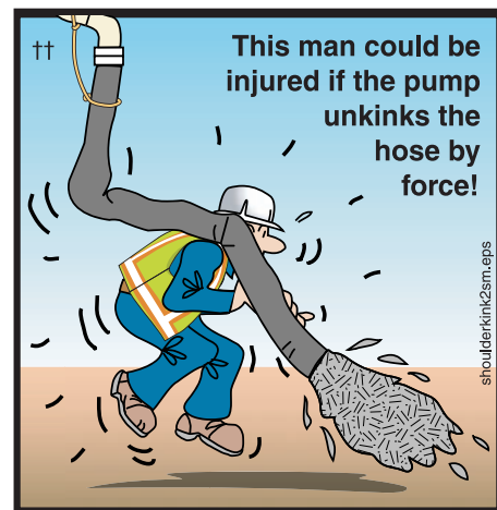
Figure 49 Kinking the hose creates a hazard
