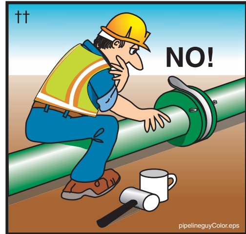
Figure 73 Never straddle or sit on a pressurized pipeline
