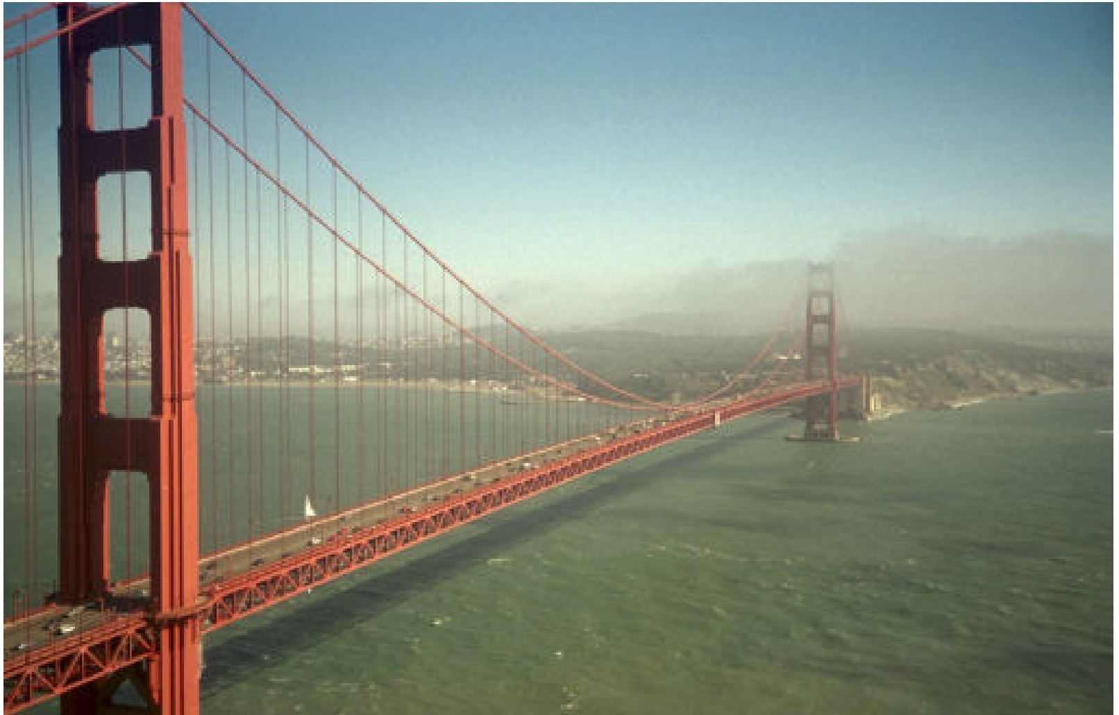
Golden Gate Bridge Project – 1930's
